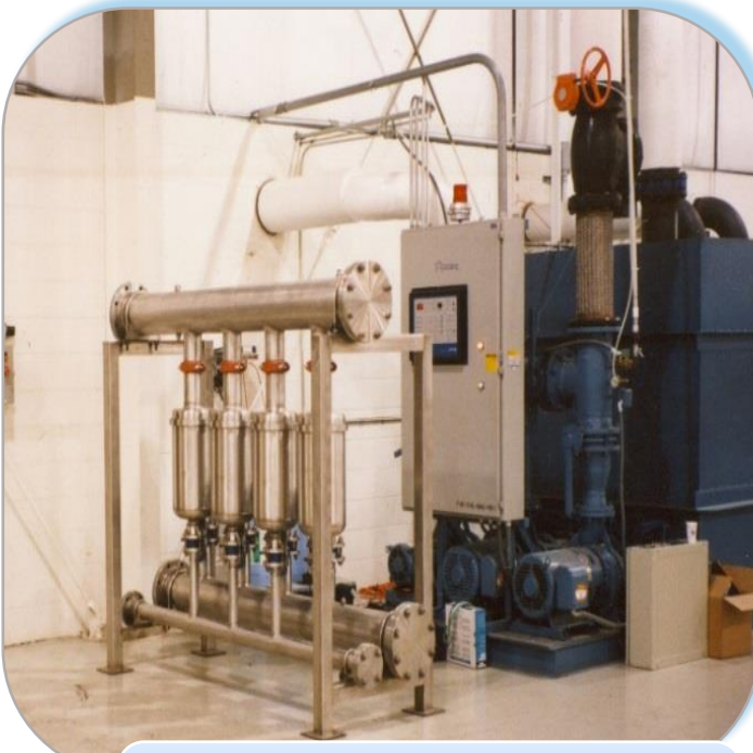
EZ Clean EC700S, 4-Pod Filter Flowrate: 1,200 gpm Filtration: 125µ Absolute Gap
