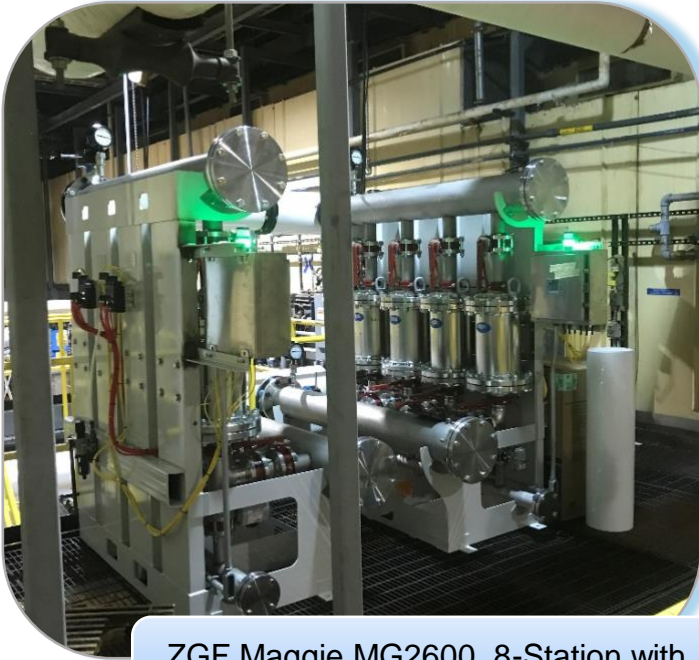
ZGF Maggie MG2600, 8-Station with Smart Drum PLUS (SD+), 2,000 gpm
