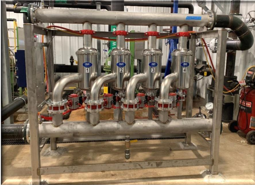
The EC700S's modular "pod" design can meet any flow requirement greater than 200 gpm. The system flowrate and level of filtration (micron rating) determines the required number of pods.
