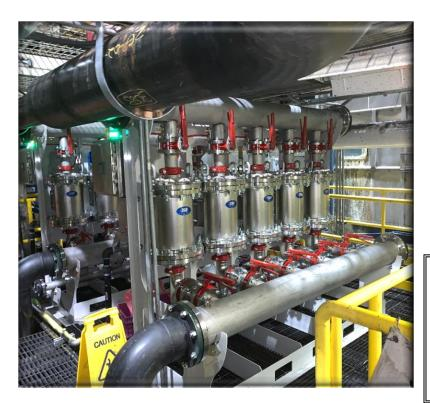
ZGF Maggie technology is a fully automatic, in-line, high intensity, self-cleaning magnetic separator. The innovative and patented Maggie is the best available technology for separating magnetic contaminants from process fluids. Maggie removes most ferrous particles 5 micron and larger and will also remove sub-micron particles without damaging critical process fluids such as machining coolants, cleaning / degreasing solutions and polymer quench fluids.
