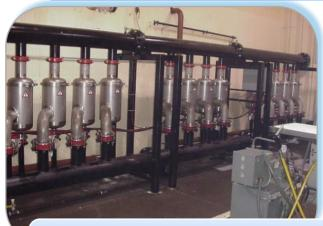
ZGF EZ CLean EC700S, 13-Pod, permanent media, fully automatic filtration system rated at 1,500 gpm
