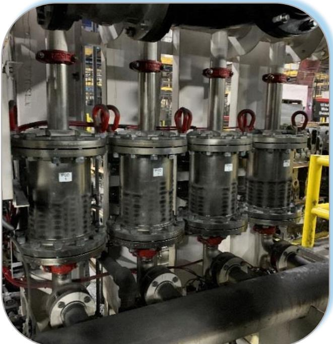
**Maggie MG2600, 4-Station, 1,000 gpm, in-line magnetic separator with Smart Drum Plus fluid recovery system**
