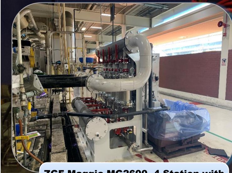
ZGF Maggie MG2600, 4-Station with Smart Drum PLUS fluid recovery system rated at 1,000 gpm
