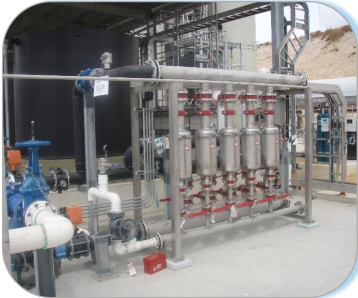
ZGF EZ Clean EC700S, 5-Pod Flowrate: 238 gpm
