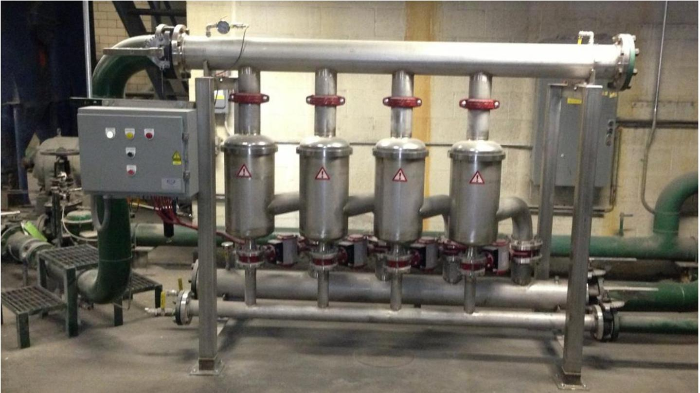
The EC700S is the most advanced, automatic, non-disposable liquid filtration system. **The EC700S's modular "pod" design can meet any flow requirement greater than 200 gpm.** The system flowrate and level of filtration (micron rating) determines the required number of pods. The EC700S is utilized to filter a wide variety of liquids including machining coolant, wash solutions, cooling / process water, waste water, and many other process fluids.
